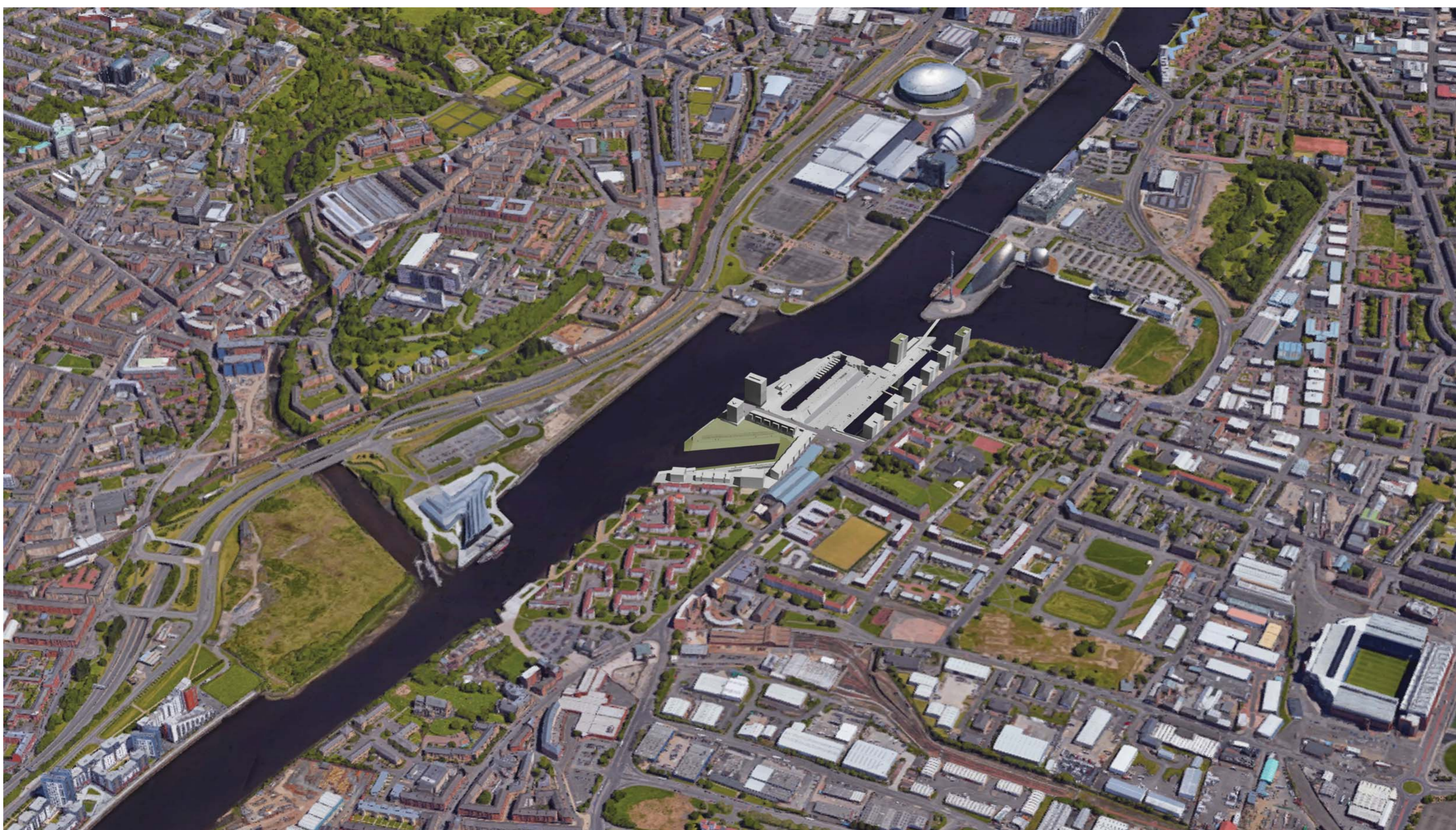
Aerial view of the Graving Docks looking North East
